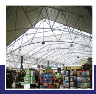
The Atrium structure at Wilson's Garden Center features curved trusses and shade cloth, allowing for natural ventilation and lower energy costs.
