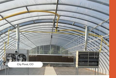
The Columbine comes as a 30' wide span and can have a peak height of up to 12'. Roll-up sidewalls are most common, but mechanical ventilation is available.
