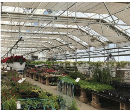
Curtain system in retail setting
