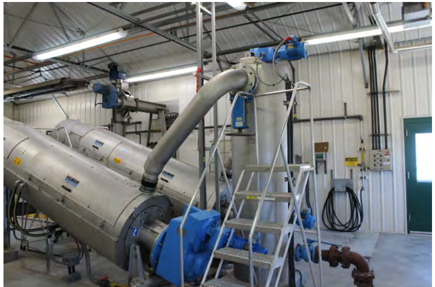
The same greenhouse frame style can be adapted with different coverings for different facility needs. Here an a-frame style structure is covered with metal decking to accommodate screw press equipment.
